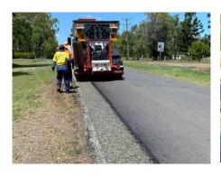
Edge break repairs are a breeze with cabin control of rotary broom stone / spray selection. Operates on both left and right hand side for increased application.
