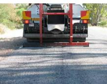
Road profile correction using full width adjustable screed bar.
